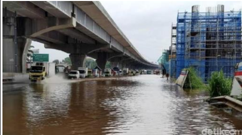
Picture 3. Flood at the Jakarta-Cikampek toll road
