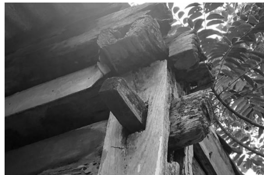
Figure 11 Cathokan system at Omah Kahar Muzakkir Source: Author, 2023
