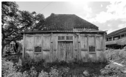
Figure 3 Kahar Muzakkir Joglo house condition in the present Source: Prihatmaji, 2013
