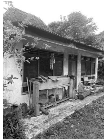
Figure 6 North elevation of Omah Kahar Muzakkir Source: Author, 2023
