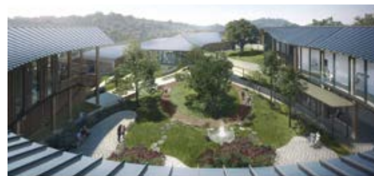
rendering of the Ohana mental health facility in Monterey, Calif., that is being constructed with cross-laminated timber in modules that can be assembled off site. BBJ
