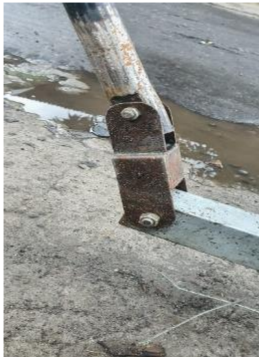
Gambar 4. 22 Flexible Joint
