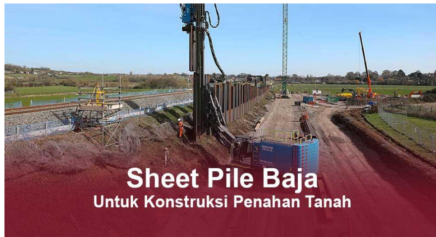
Gambar 3. 7 Revetment Turap Baja
