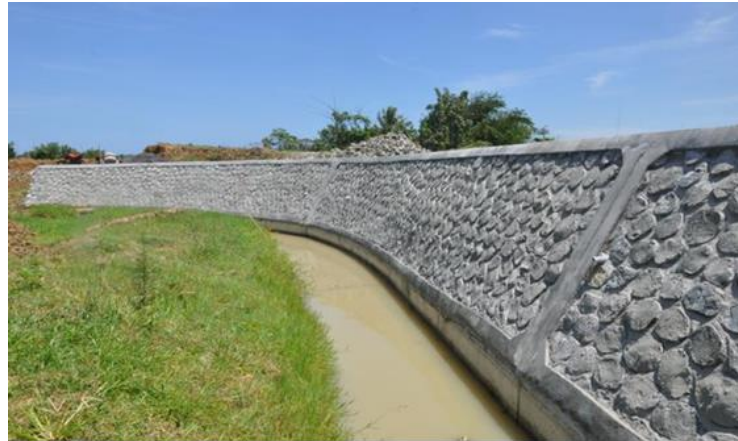
Gambar 3. 10 Revetment Pasangan Batu
