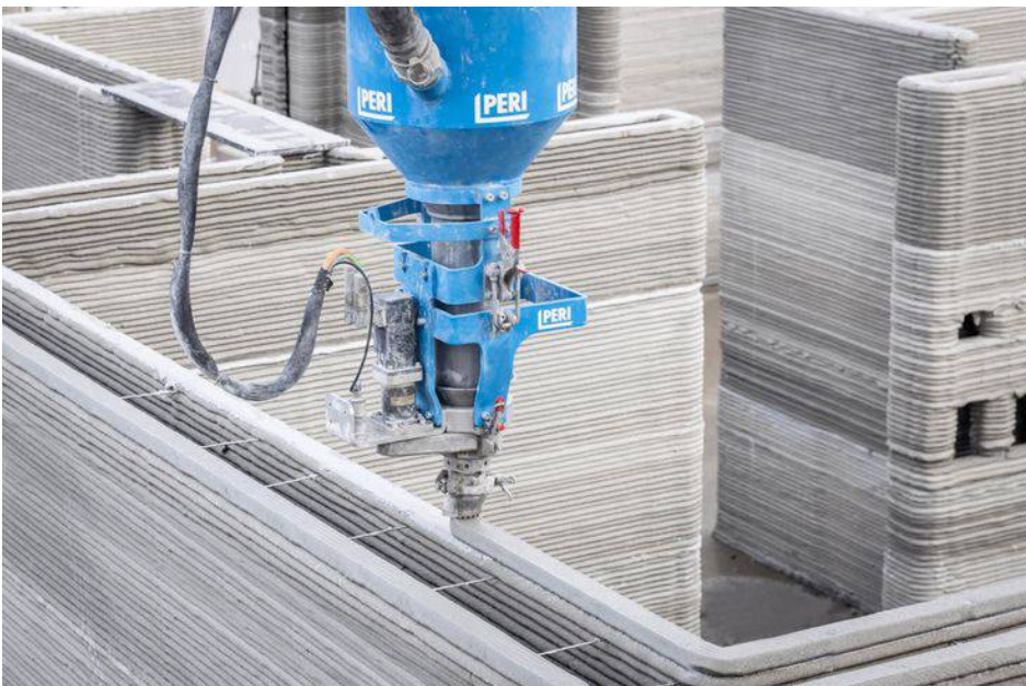
Figure 1.5 3D print construction (Source: printtimber.org)
