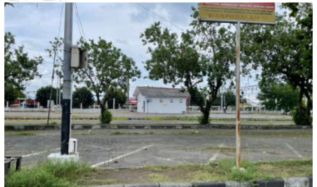
Figure 1.4 Adisutjipto airport parking facility
