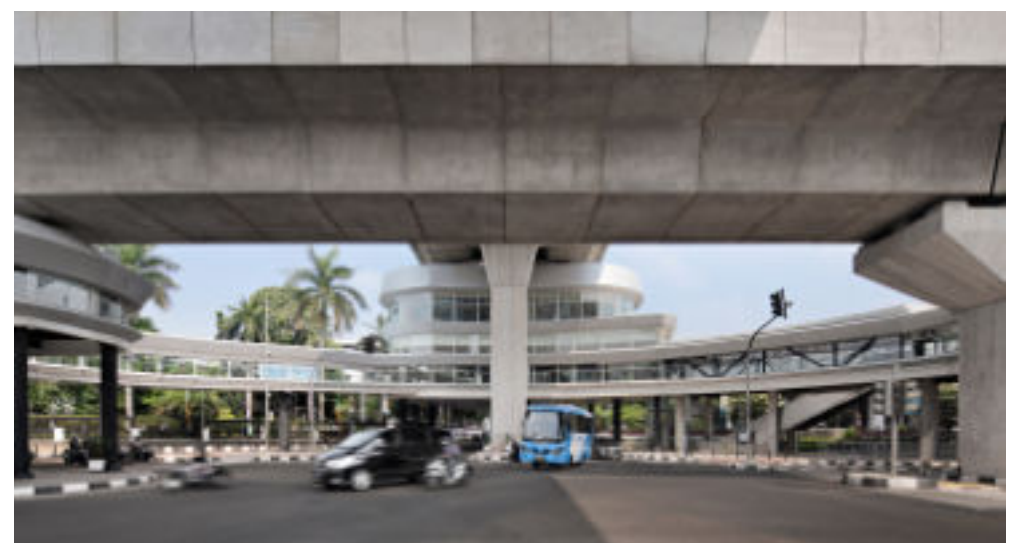
Figure 2.32 CSW from street level
