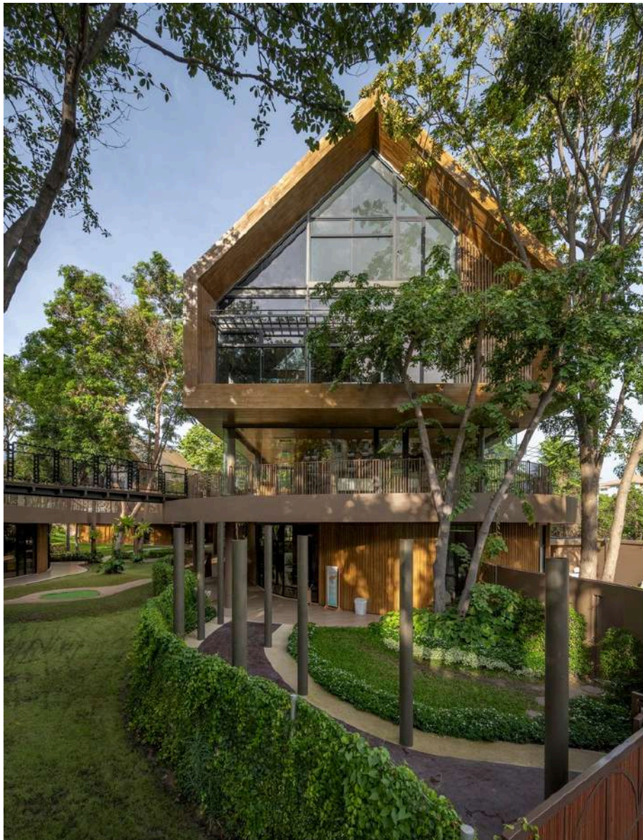
Figure 2.23 Lovell International School Source: Archdaily, 2023
