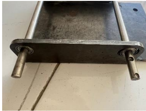
Gambar 4- 4 Pemasangan Besi AS ke Base Conveyor
