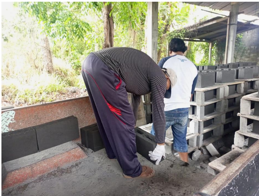
Figure 4.6: The worker is moving the concrete brick
