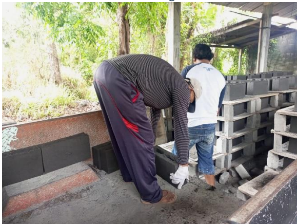
Attachment 43: Worker lifts the concrete brick into the pickup car
