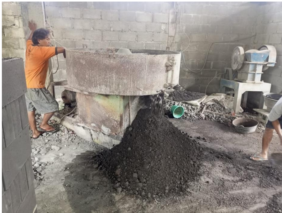
Figure 4.4 :The cement paste is out from the mixing machine
