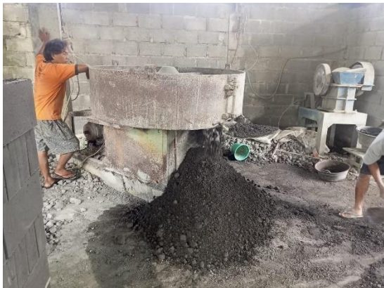
Attachment 5: The mixer is pouring out the cement paste
