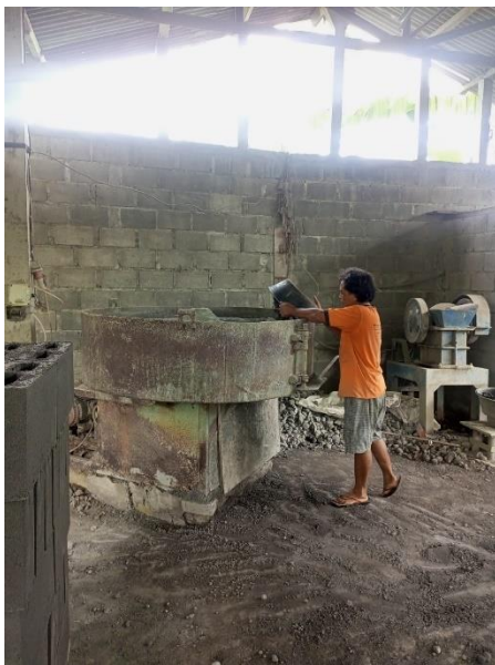
Attachment 3: Worker pouring sand into mixer
