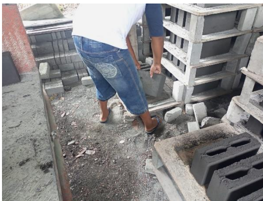
Attachment 41: The worker lifting the undried concrete brick
