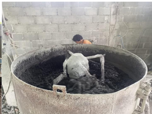
Attachment 11: The worker is pouring sand into mix machine Attachment 12: The mix machine is mixing
