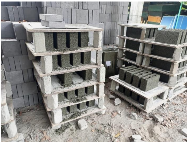
Attachment 33: Drying concrete brick
