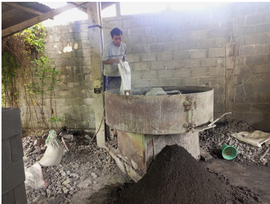
Figure 4.2: Worker is pouring the cement
