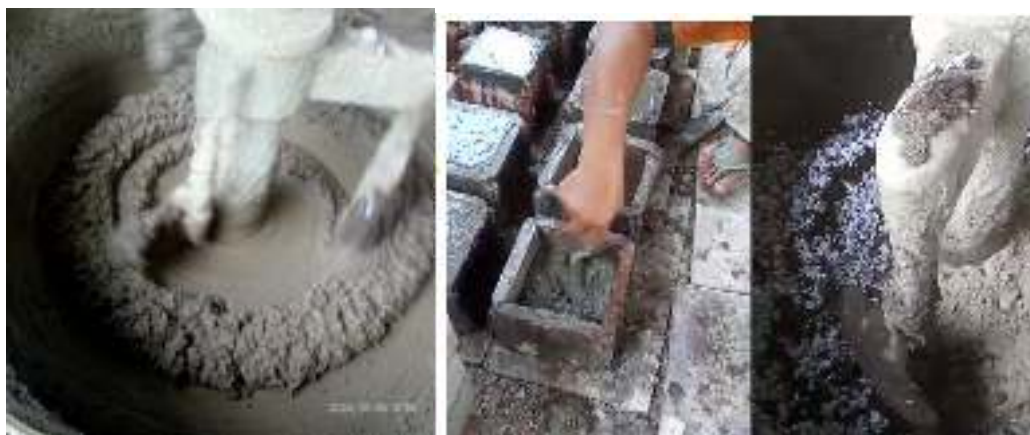
Figure 4.4 Mixing and pouring the mixture into the moulds
