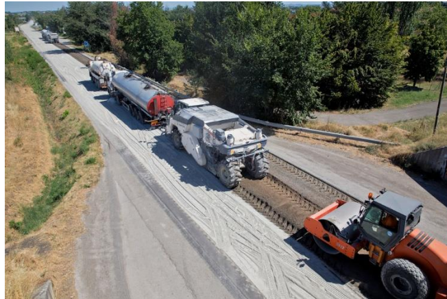
Gambar 3.41 Cold Recycling
