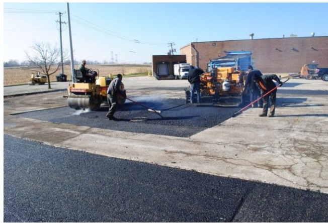
Gambar 3.35 Full-depth patching
