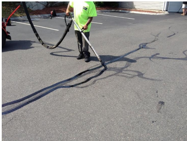
Gambar 3.34 Crack Sealing
