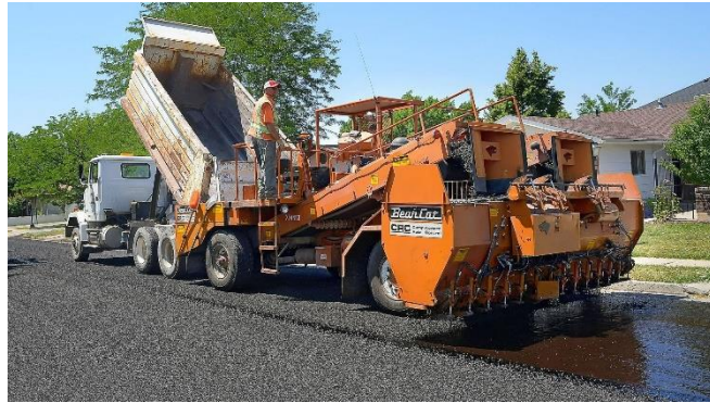
Gambar 3.39 Chip Seal
