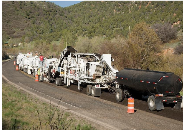
Gambar 3.44 Cold In-Place Recycling
