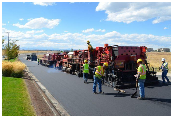
Gambar 3.43 Hot In-Place Recycling
