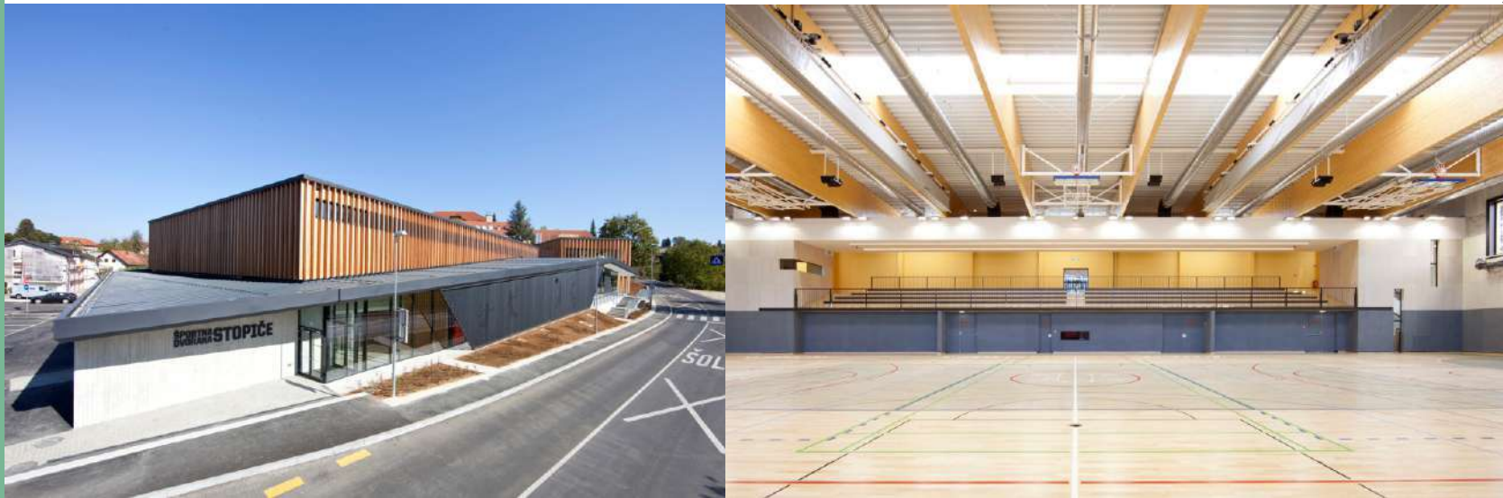
Figure 2.10 : Sports Center Stopiče . Source : ArchDaily
