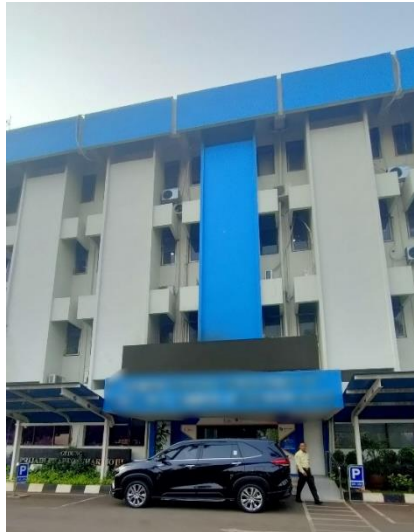
Figure 3 Directorate General of ABC of Ministry XYZ's Building
