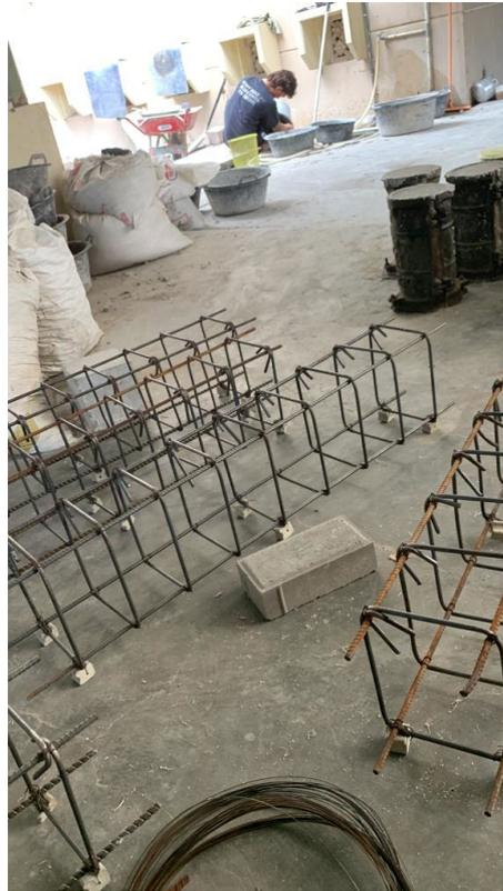
**Gambar L-7.1 Perakitan Tulangan**
