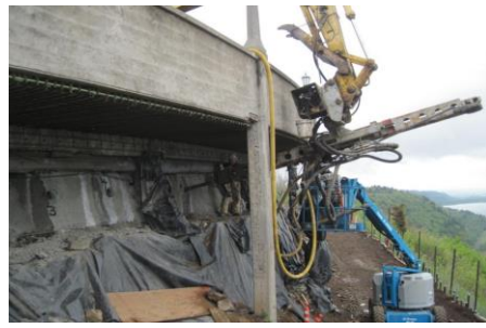
Figure 3.8 Nail Holes Drilling
