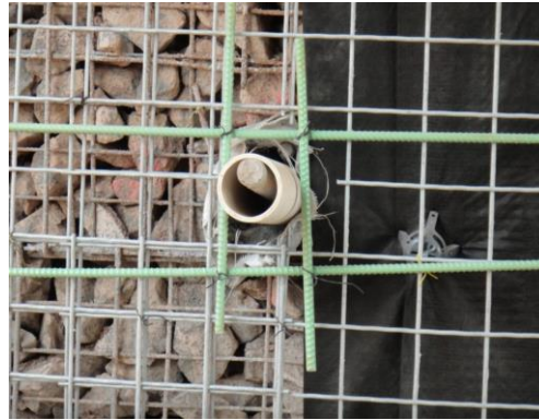
Figure 3.10 Shotcrete Reinforcement
