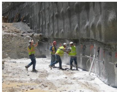
Figure 3.9 Nail Bar Installation
