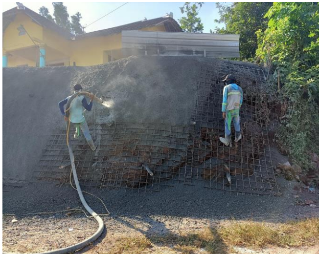
Figure 3.5 Shotcrete Installation
