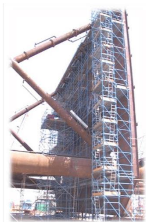
Gambar 3. 5 Access Tower Scaffold
