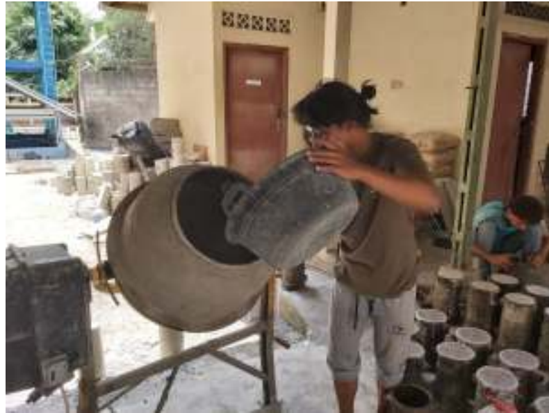
Lampiran 6.6 Proses Mixing Campuran Beton
