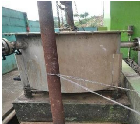
Gambar 2.6 Unit Stone Trap
