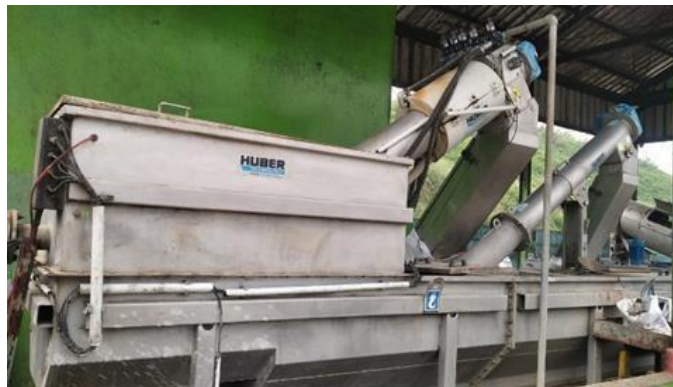
Gambar 2.8 Unit Sludge Acceptance Plant
