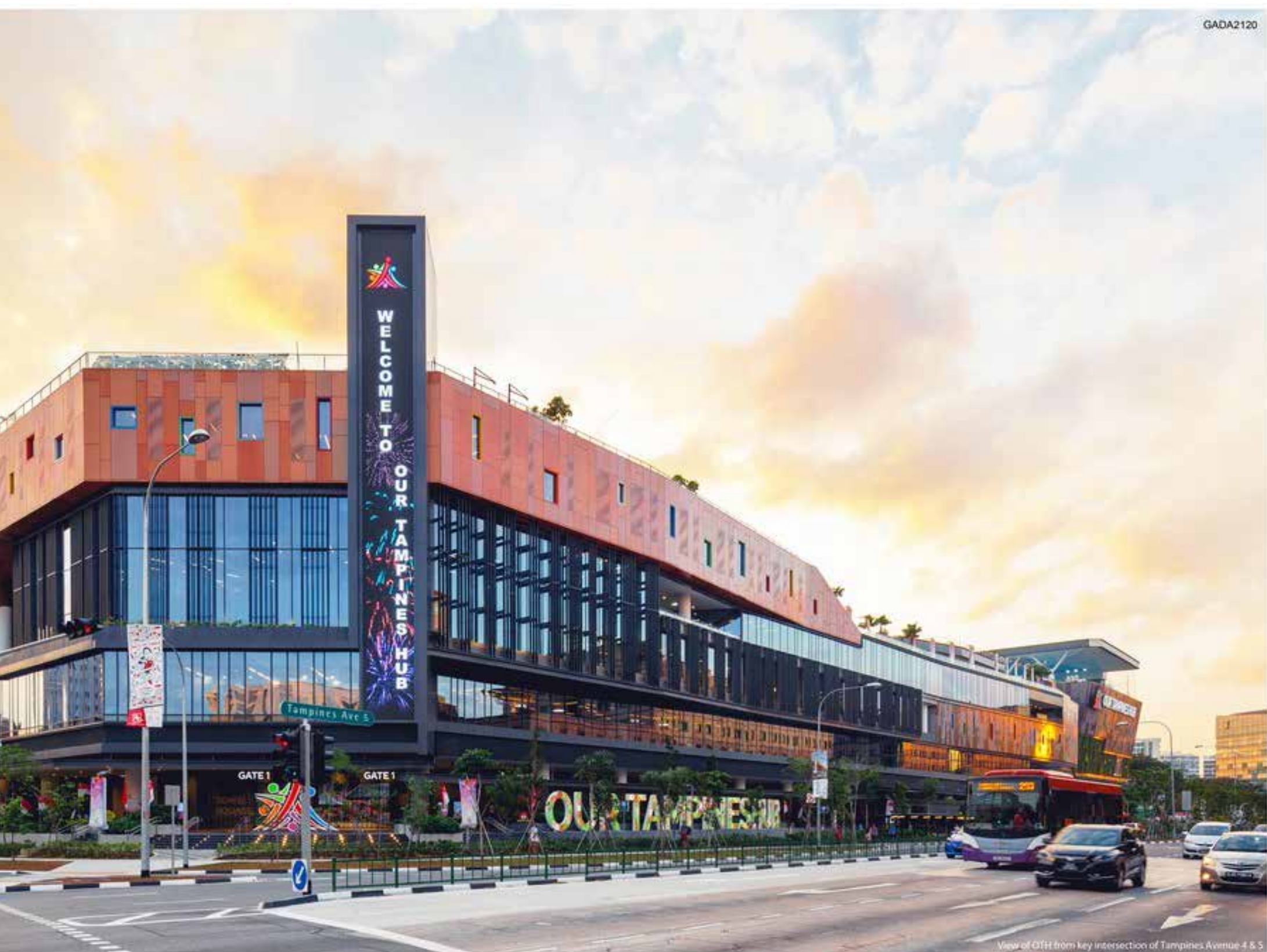
View of OTH from key intersection of Tampines Avenue 4 & 5
