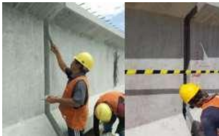
Gambar 5.18 Pengolesan lem epoxy adhesive Sumber: PT.PP Persero (Tbk)
