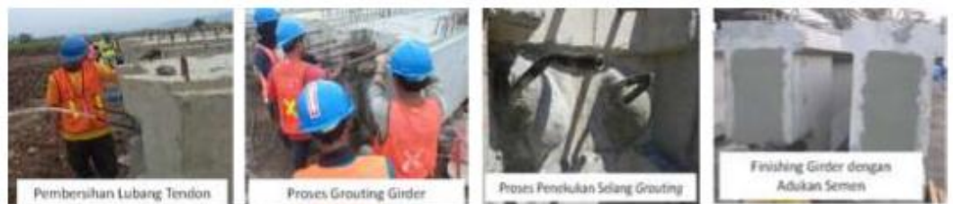
Gambar 5.21 Grouting Girder Sumber: PT.PP Persero (Tbk)
