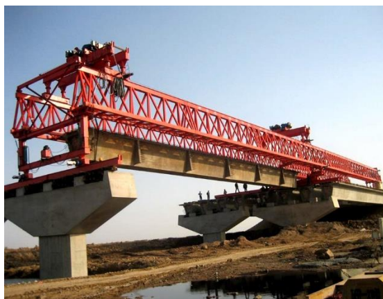
Gambar 3.10 Launcher Gantry Sumber: Google.com
