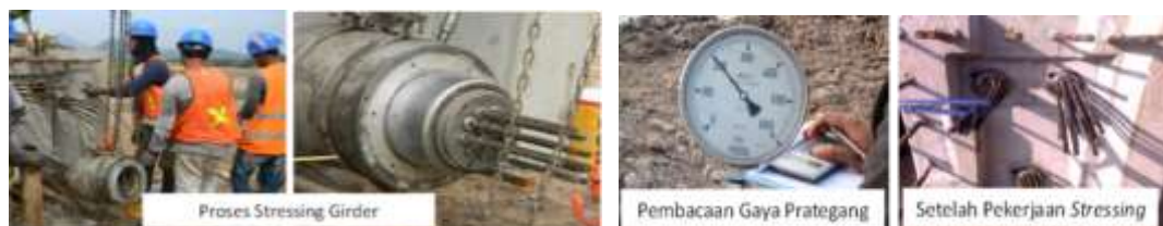
Gambar 6. Stressing Girder
