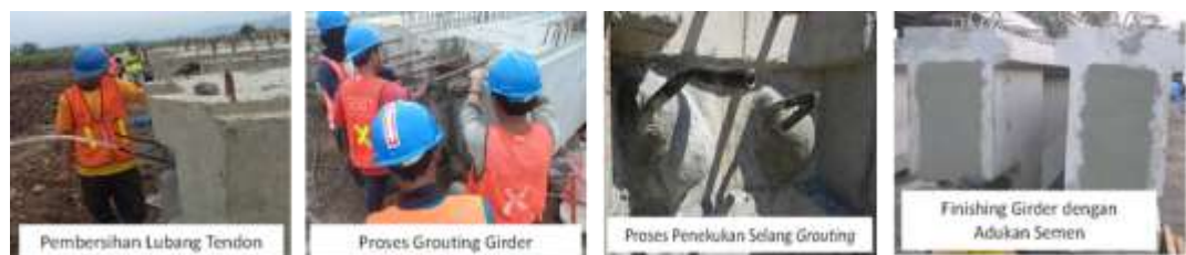
Gambar 7. Grouting Girder
