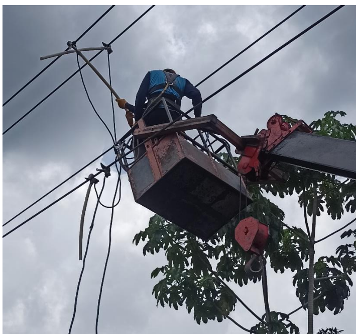
Gambar 5.1 Pemasangan ground cluster
