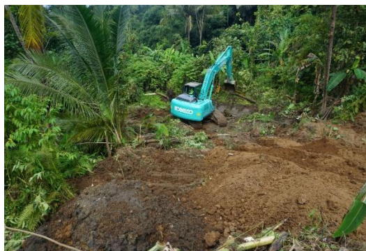
Gambar 5.19 Clearing dan Grubbing
