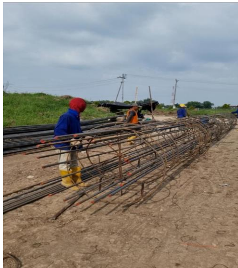
Figure A-1.2 Reinforcement Steel Fabrication
