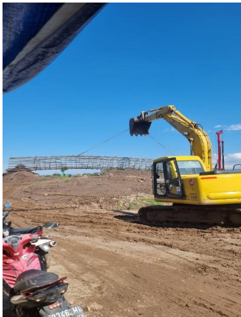
Figure A-1.7 Transfer of reinforcement steel to hole location
