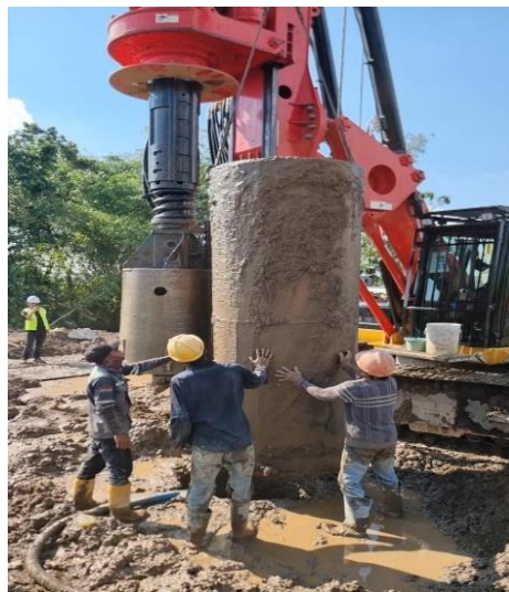
Figure A-1.4 Casing Installation at Ground Drilling Points
