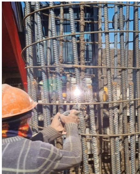
Figure A-1.8 Reinforcement Steel Connection
