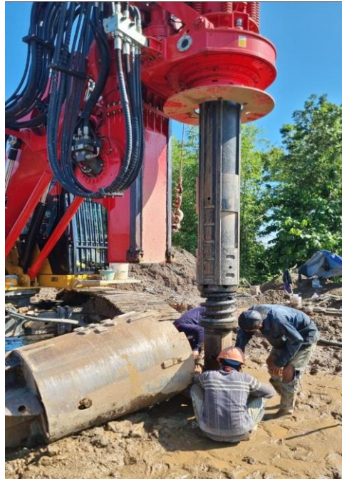
Figure A-1.1 Setting the borepile Wash Boring
