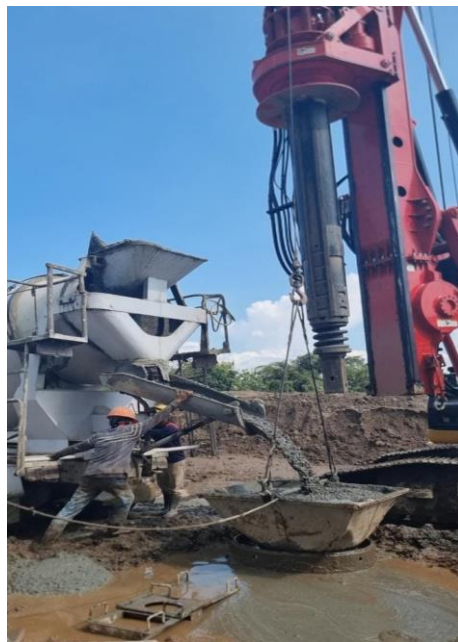
Figure A-1.10 Bore Pile Foundation Casting Process
