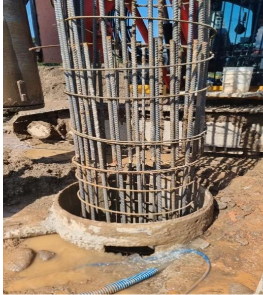
Figure A-1.8 Installation of the Bore Pile Reinforcement to the Hole
