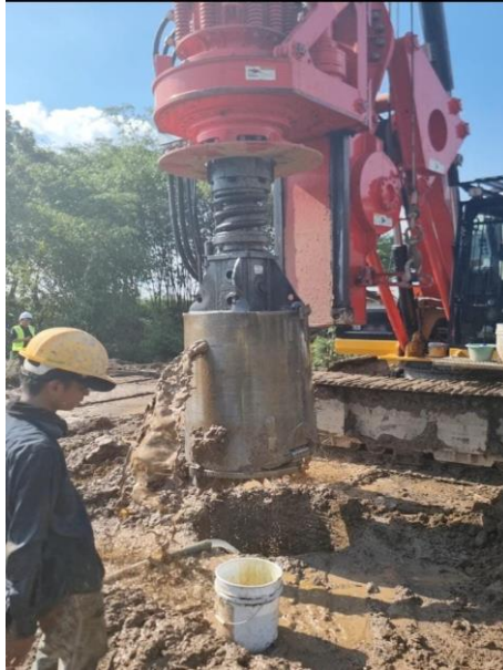
Figure A-1.3 Initial Drilling Point
