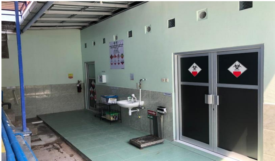
Gambar 4.9 Tampak Depan TPS RS Condong Catur
