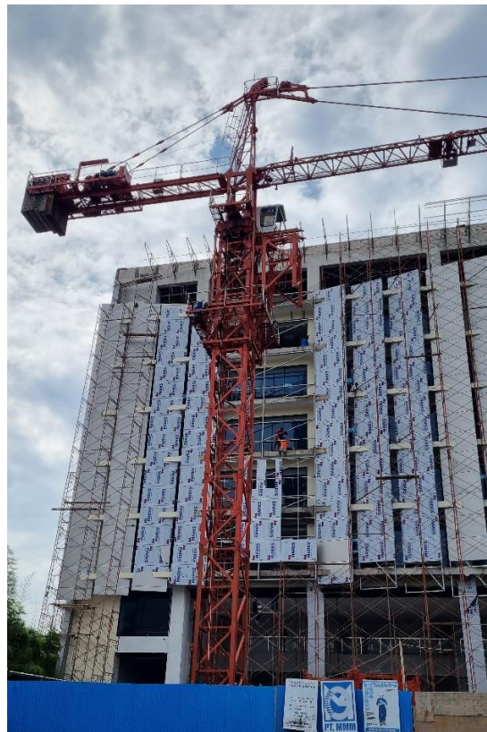
Figure A-1.4 Demolition of Mast Section of Tower Crane
