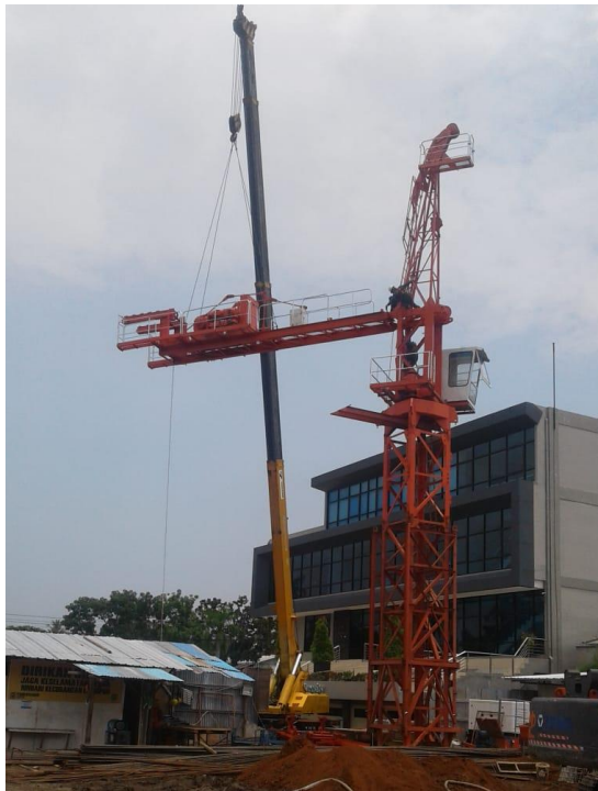
Figure A-1.3 Installation of Counterweight of Tower Crane
