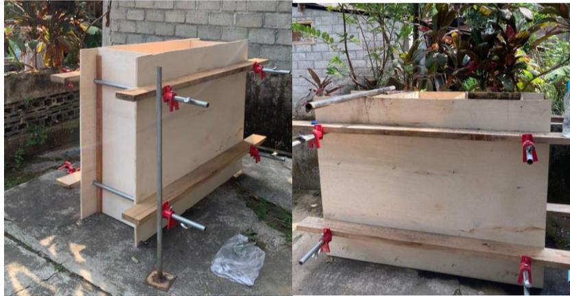
**Gambar 1** Bekisting dinding tanah
