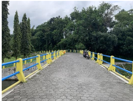
Gambar A6. View Jembatan
