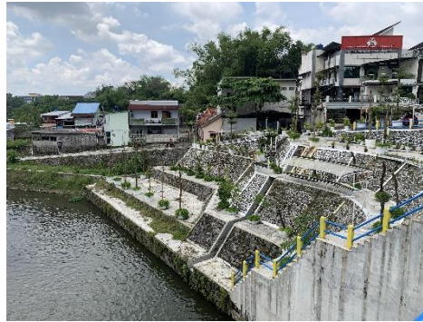
Gambar A9. View Dinding Penahan Tanah
