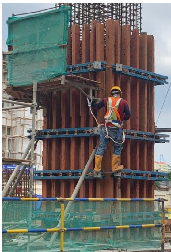
Gambar 3. 2 Bekisting Semi Sistem
