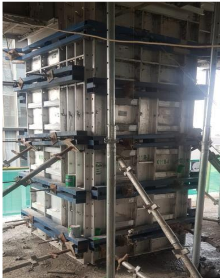
Gambar 3. 4 Bekisting Aluminium (Sumber: PT PP (Persero) Project Planning Presentation )
