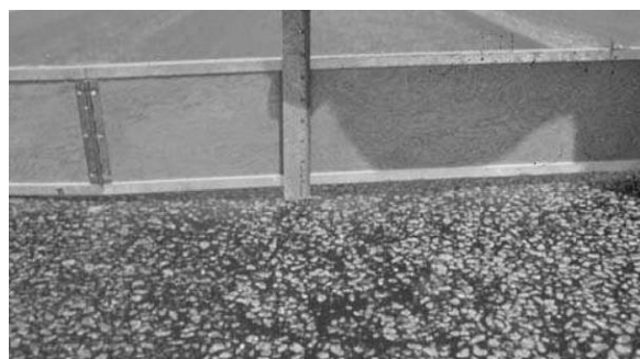
Gambar 3.14 Alur ( Rutting )
