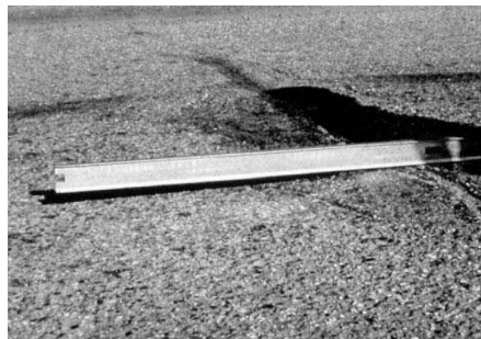
Gambar 3.8 Cekungan ( Bumps and Sags )
