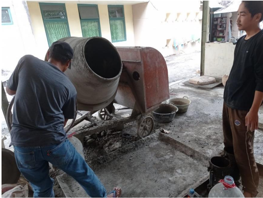
Gambar L-2.5 Proses Mixing Campuran Beton
