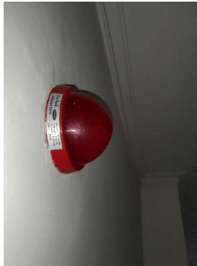
**Gambar L-4** *Fire Alarm Indicator*
