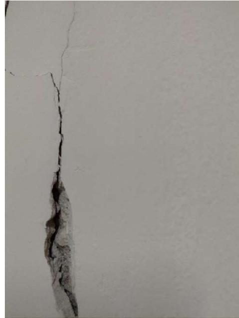
**Gambar L-20 Dinding Retak**
