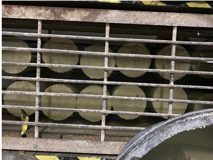
Gambar L8.5 Proses Curing Beton
