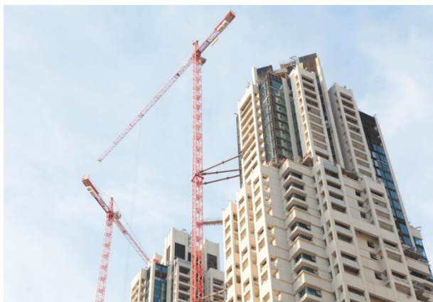
Gambar 3.4 Tied in Crane
