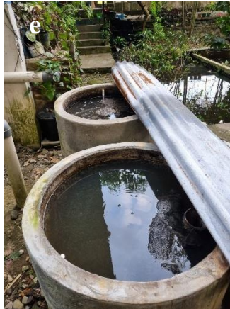
Gambar 4. 1 (a)inlet, (b)manhole ABR, (c)Anaerobic Baffled Reactor, (d)Rotating Biological Contactor, (e)unit filtrasi
