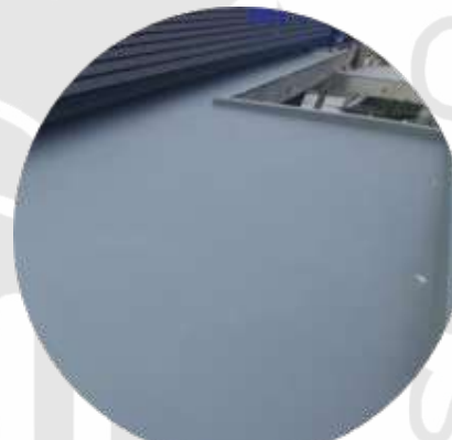
Atap Dak Beton
