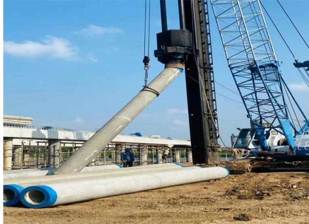
**Gambar 3. 3 Tiang Pancang Beton Precast**
