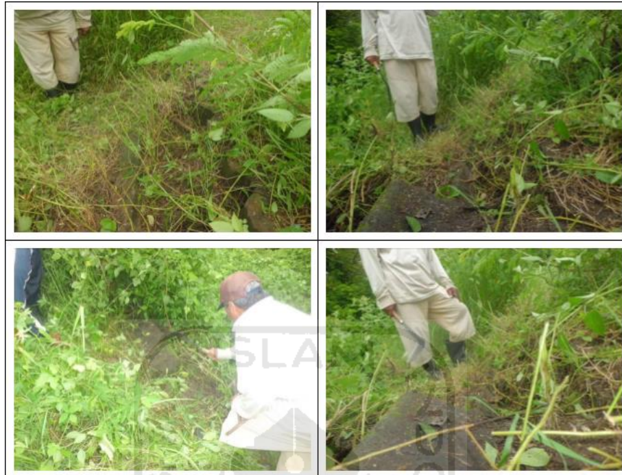
Gambar 1.4 Pecahan/Lepasan Penahan Samping Lapisan Grass Block
