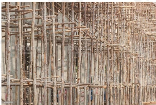
Gambar 3.11 Scaffolding Kayu/Bambu (Sumber: Peangdao, 2014)
