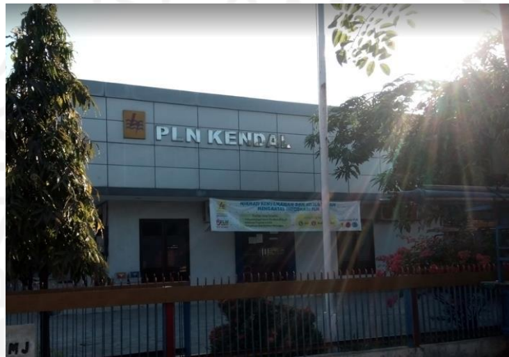
Figure 4.1 PT. PLN ULP Kendal Office
