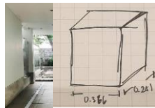
Image 20 and 21 Reinforced concrete Column, Square-shaped in Senja Coffee and Memories
