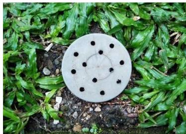
**Gambar 2.** Lubang biopori
