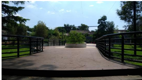
Figure 19. Fence on the brodge
