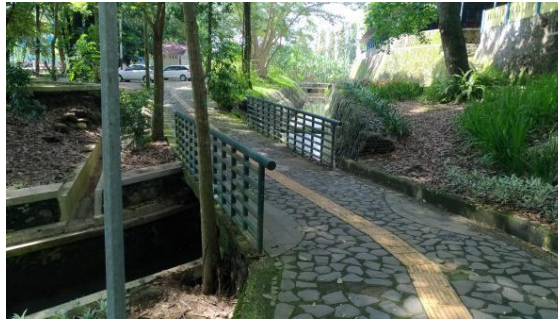
Figure 15. River bridge with blind track
