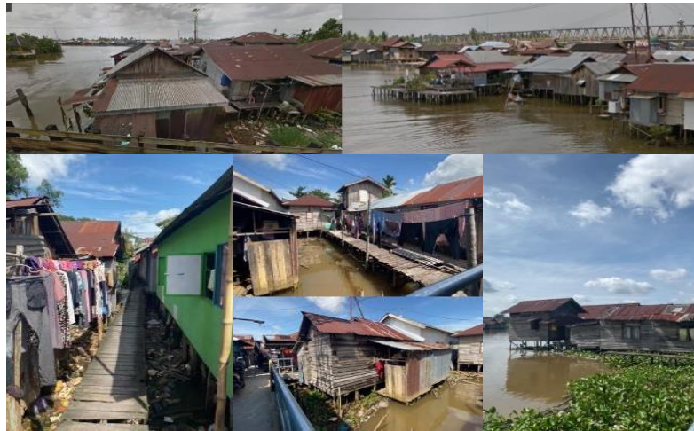
Figure 2. Condition of the target area
