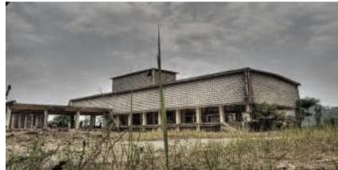
Figure 1. The condition of Abandoned Citronella Distilled Factory.
