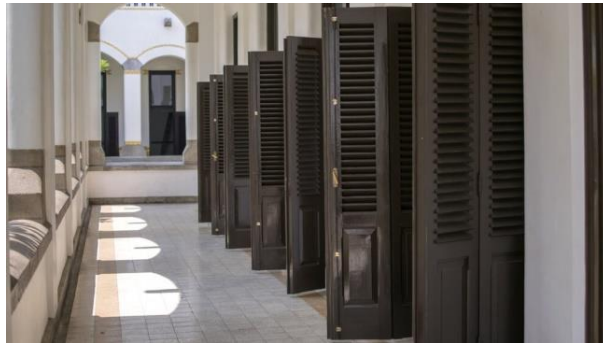
Fig 2 Lawang Sewu Outdoor Hallway
