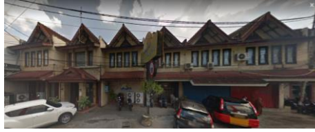
Gambar 10. Tampak Toko Sumber : Google Street View
