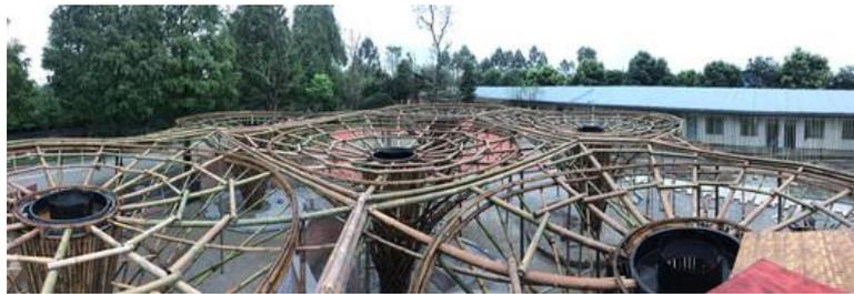
**Gambar 15** Kerangka Atap *The Bamboo Garden*
