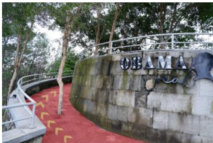
Figure 6. Provision of ramp completed with railing guard in Puncak Becici
