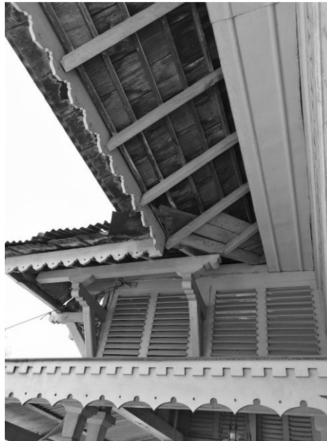
Image 7 Upper console in veranda of KGPH Dipokusumo's Residence
